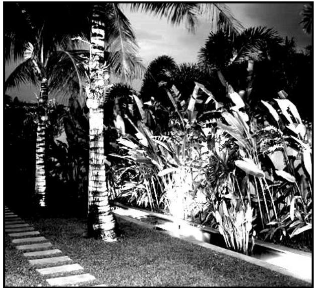
Low-voltage exterior lighting
