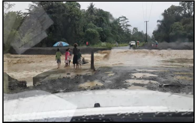
Damages by cyclone in Milne Bay province
